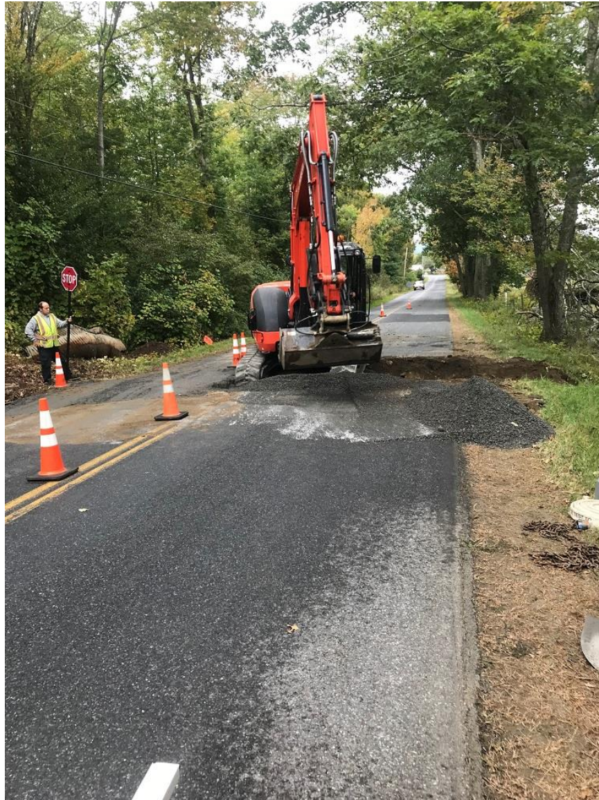
The crew changing a culvert on North Union Rd.
