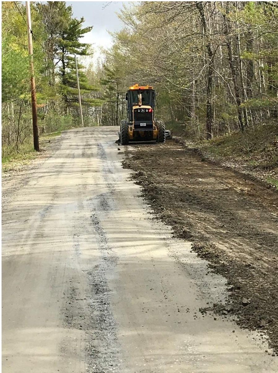
Grading Barrett Hill Road
