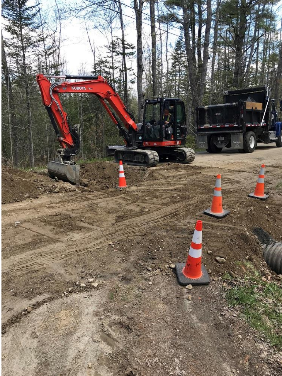
Replacing culvert on Sidelinger Rd
