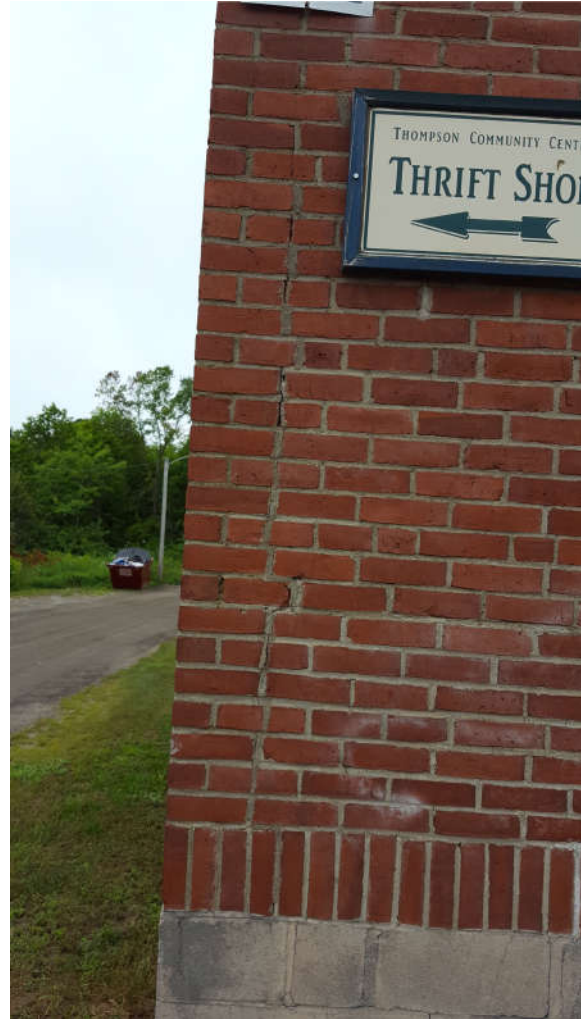
Photo 10 – Corner cracking 2018
