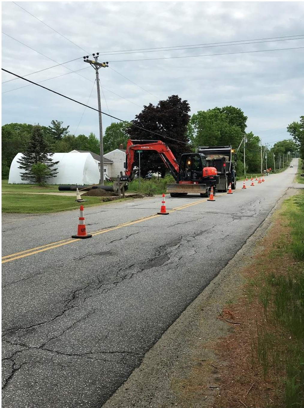
Replacing a culvert on Sennebec Rd
