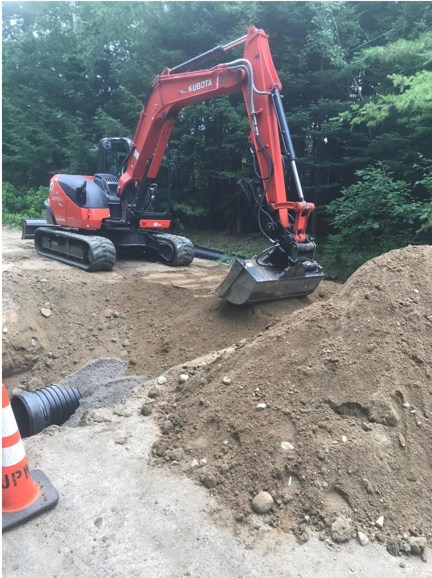
Replacing a culvert on Happy Hollow Rd
