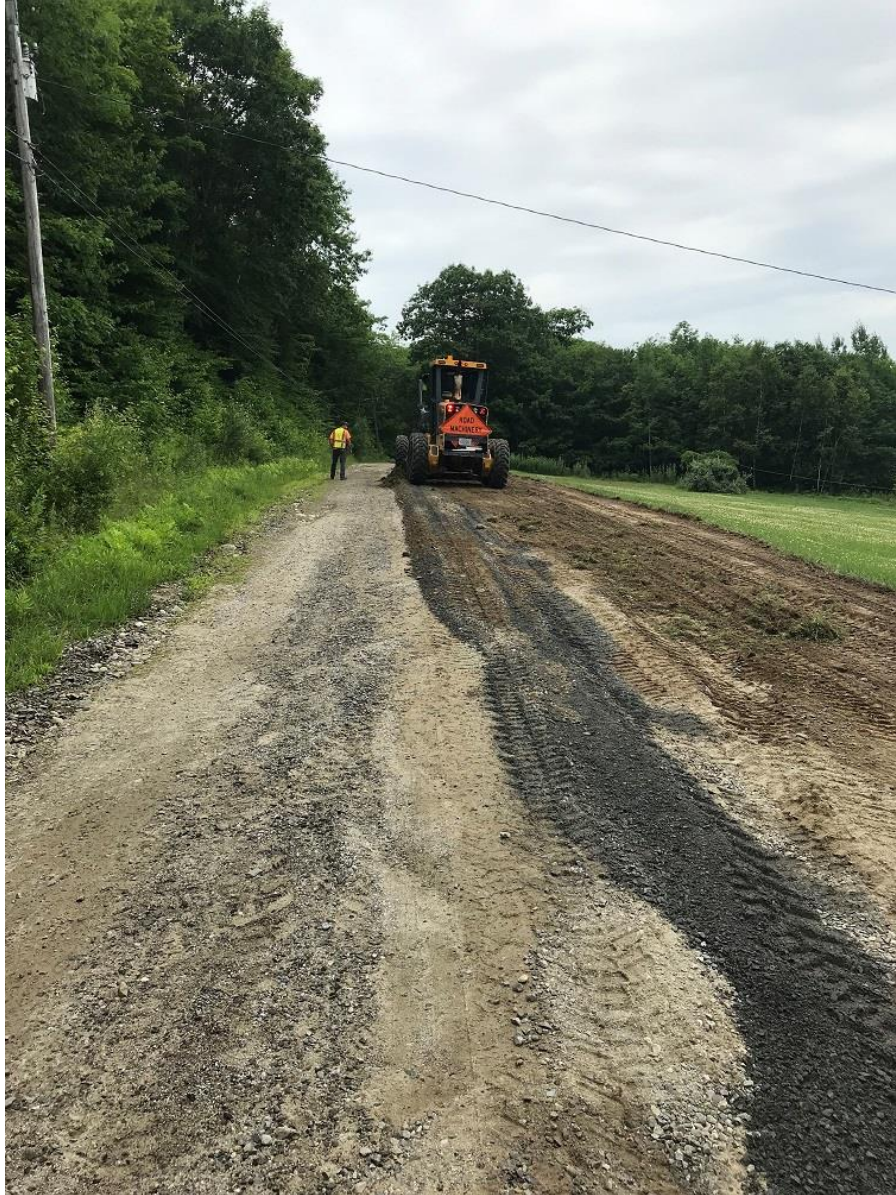
Repairing a washout on Coggins Hill
