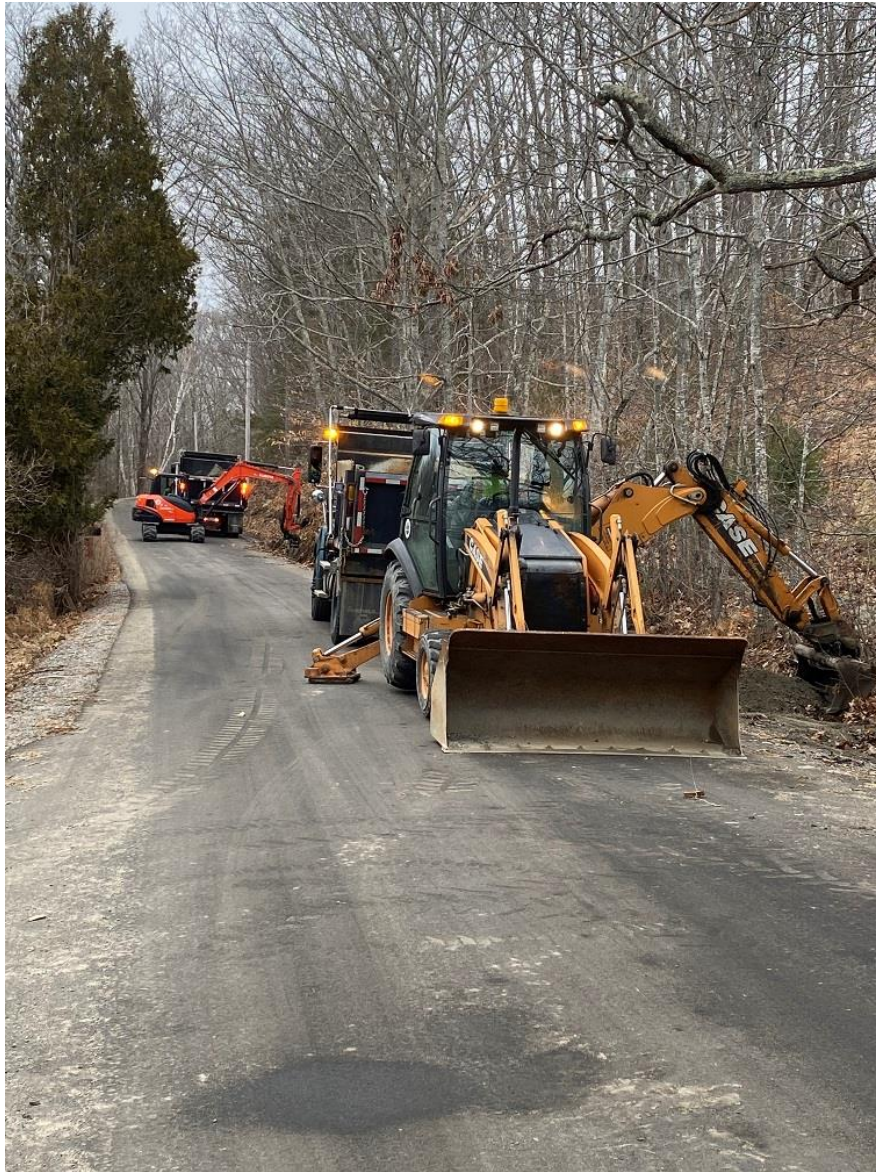
Repairing the washout on Rabbit Farm Rd
