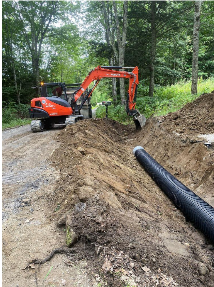
Putting in a new driveway culvert on Robbins Rd
