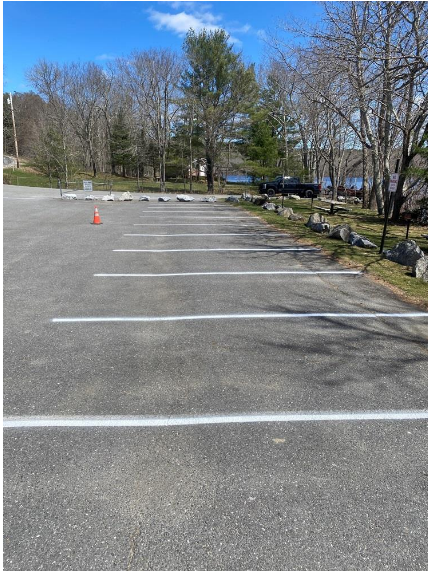
Freshly painted parking lines at Ayer Park
